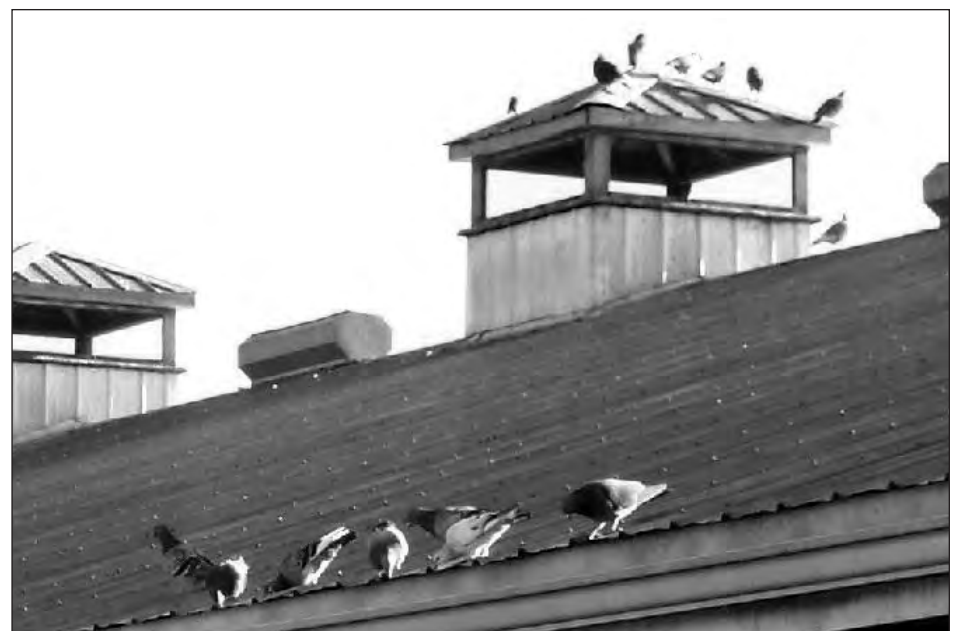
Pigeons on the Kellogg Dairy Center's roof.
