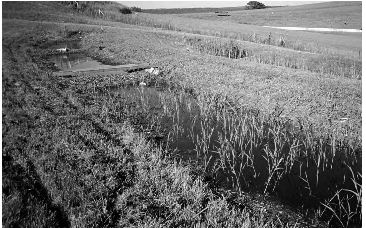
Photo of middle cells of the constructed wetland showing young Phragmites plants and rock berms separating sub-cells. The plank bridging the cell is used as a platform from which to harvest the Phragmites .
